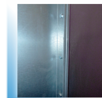
5/16" bolts with serrated lock nut
