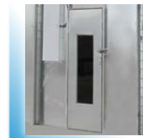
Windowed personnel access doors
